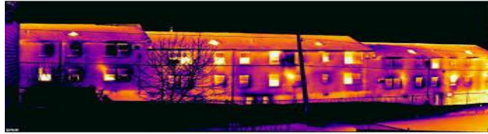
a) Infrared Image
